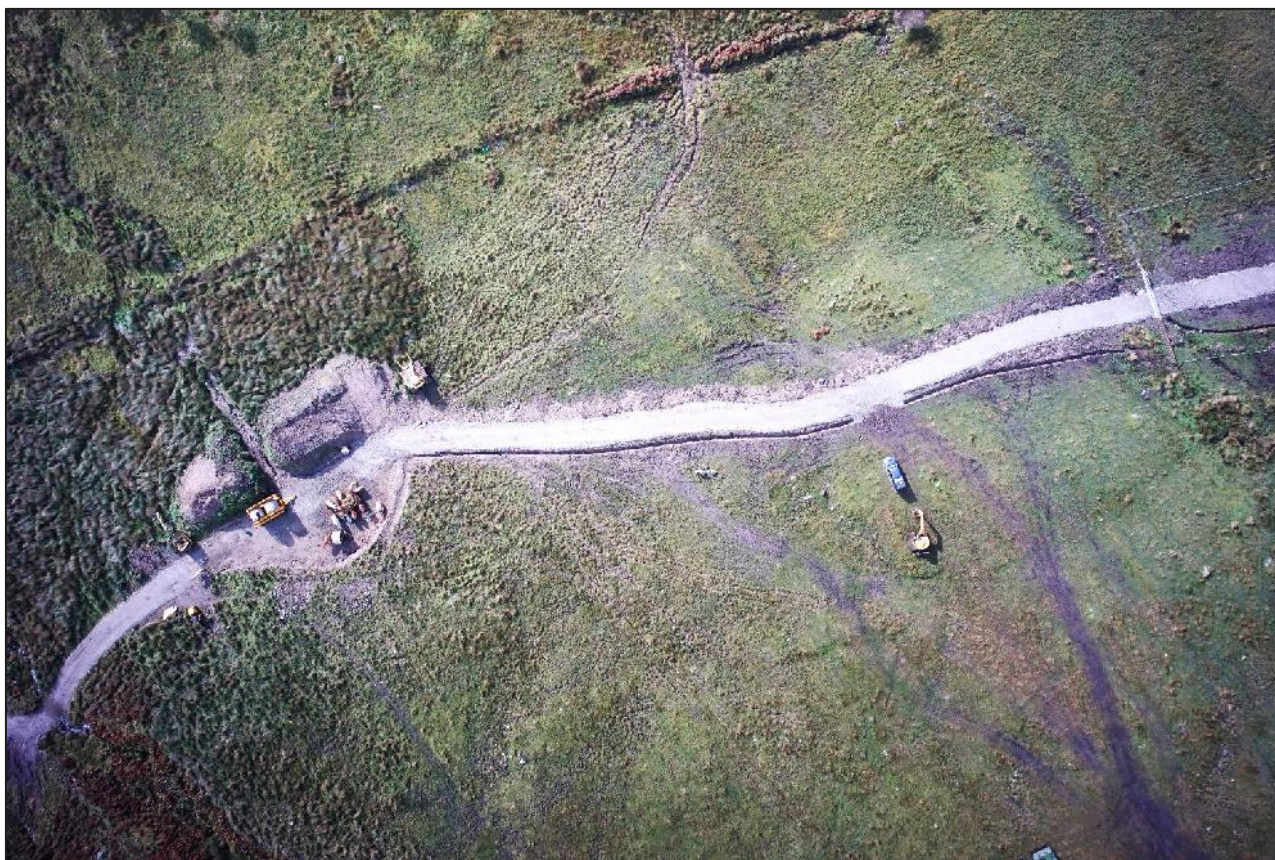
Figure 5.4: Reinstatement of cable trench adjacent to access track – aerial survey
