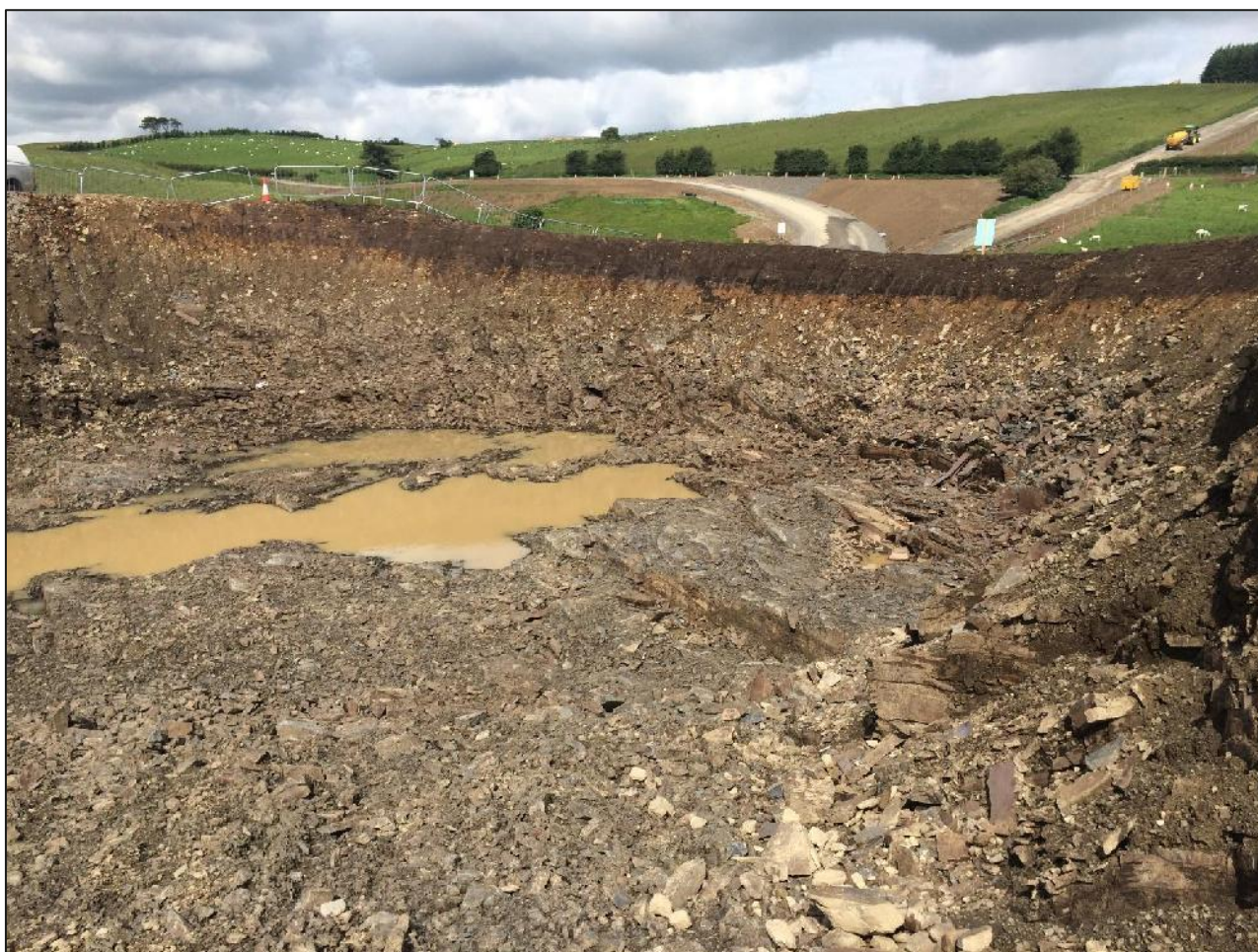
Figure 5.5: Excavated material stockpiled around the perimeter of the foundation excavation
