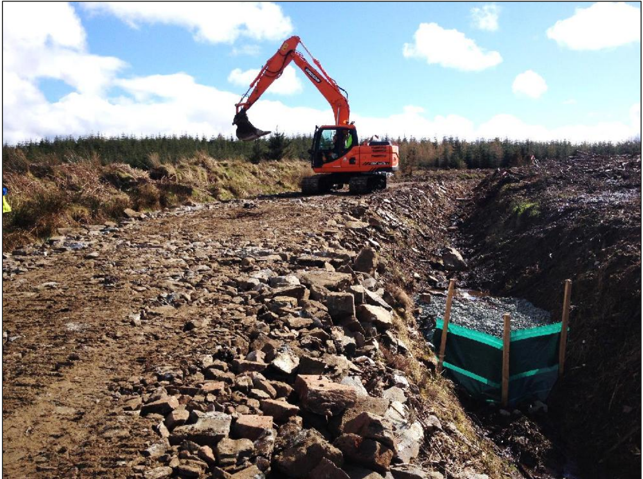
Figure 5.2: Example of verge reinstatement ongoing with drainage provision
