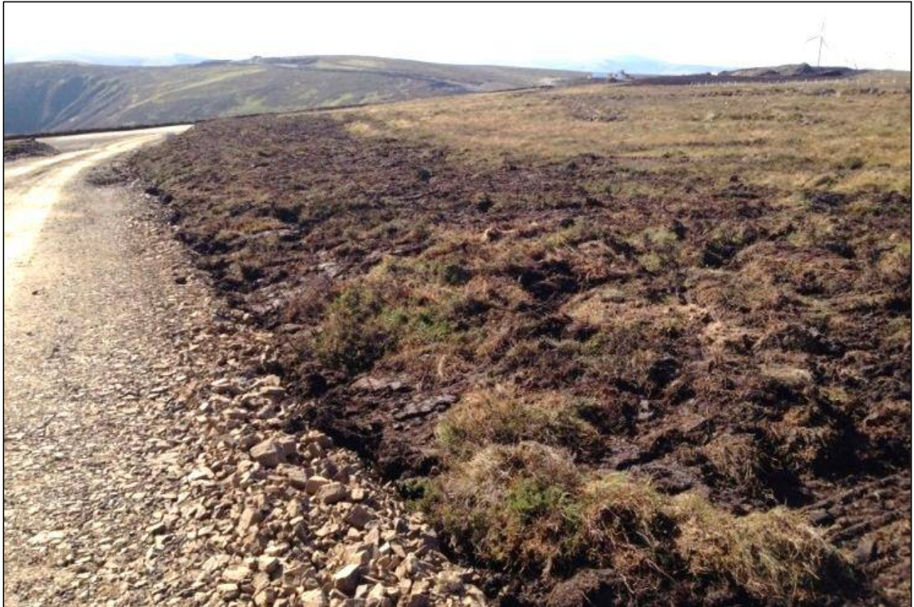
Figure 5.3: Example of access track verge reinstatement
