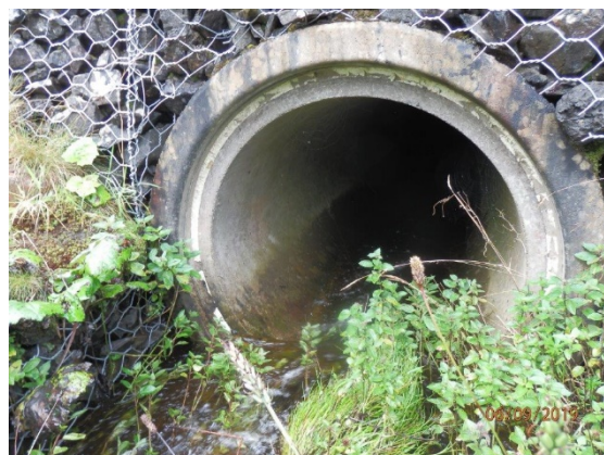
Plate 9.2: Flisk tributary - long culvert 40m downstream of Site boundary
