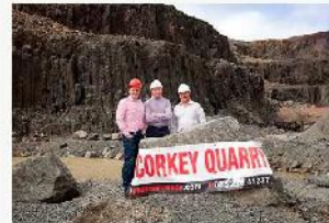
Donlan Keenan (E. Keenan & Sons), with Fergal Duffy (RES Construction Manager) and Noel Usherin (RES Construction Site Manager) during the construction of Altavaheen Wind Farm
